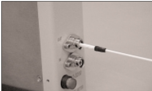
Figure 6. Cleaning bulkhead connectors
